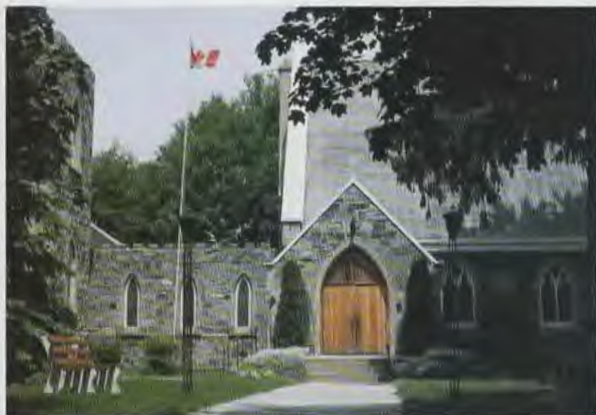
Installed in Meaford's Christ Church Anglican and dedicated to the parish's war dead, the windows contain some of the oldest stained glass in North America.
